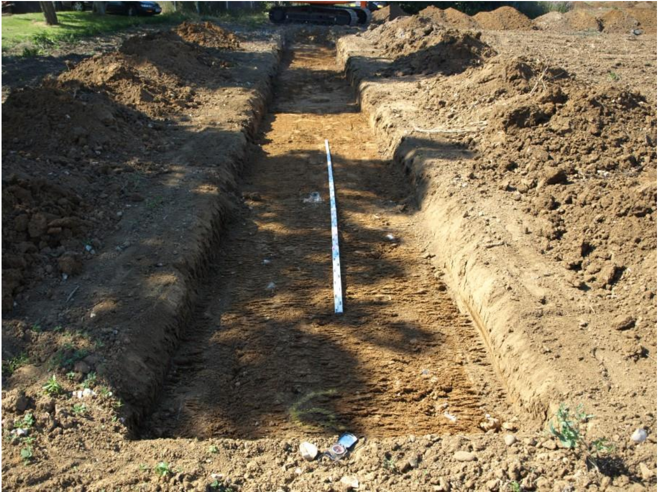
Plate 10: Looking north west at trench 6
