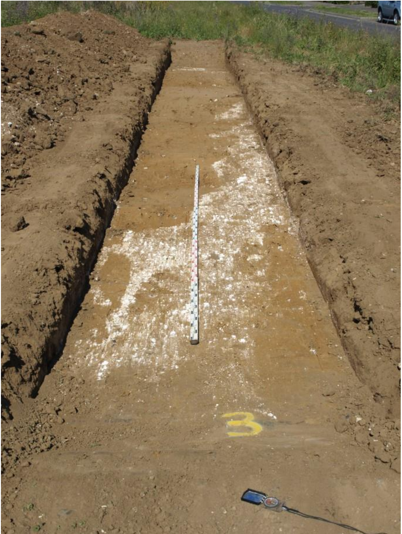
Plate 7: Looking north-east at Trench 3 with exposed modern ditch [303]
