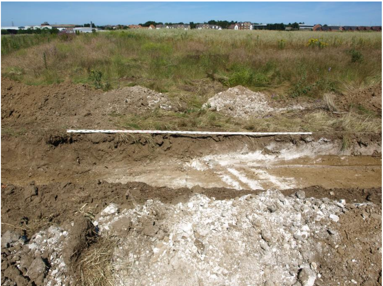
Plate 27: Looking north east at section through build up ground exposed in Trench 20 – middle. Visible chalk is a modern redeposit indicating edge of hollow/quarry approach.
